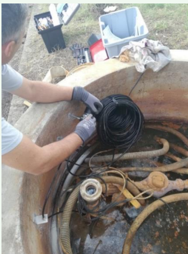
Figure 2: Brackish water is continuously monitored for electroconductivity, temperature and flow.
